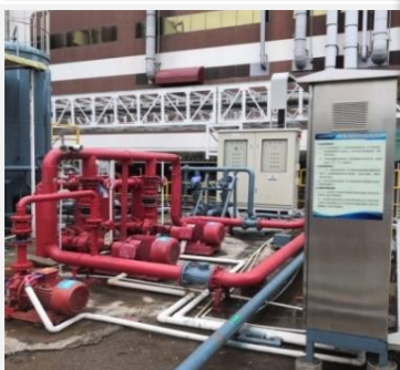
Open-air fire pump room (after improvement)
