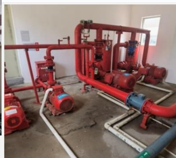
Installation of a spare booster pump (after improvement)
